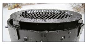
Left: A Teton Raptor Center vent screen. The Poo-Poo Project's goal is to prevent wildlife entrapment within vent pipes without compromising ventilation by installing these screens across the U.S.
