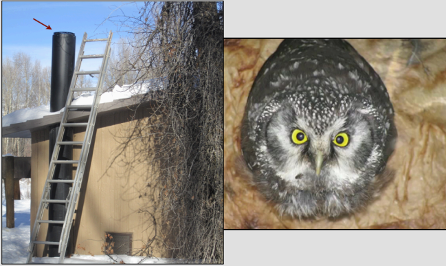
The screens cover the open vent pipe (marked with a red arrow, left) to prevent owls from entrapment, like this Boreal Owl that was rescued from a vault toilet in Boise National Forest. Owl photo: USDA Forest Service.
